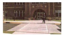
Traffic calming devices such as a raised crosswalk help illuminate the pedestrian crossings and slow motor vehicle traffic.
