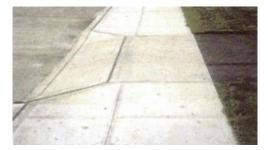
Driveways should be designed so the sidewalk continues through the driveway in a relatively flat and level alignment.
