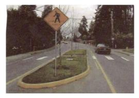
A road diet, such as the one above, may decrease motor vehicle speed and reduce the number of lanes a pedestrian must cross.
